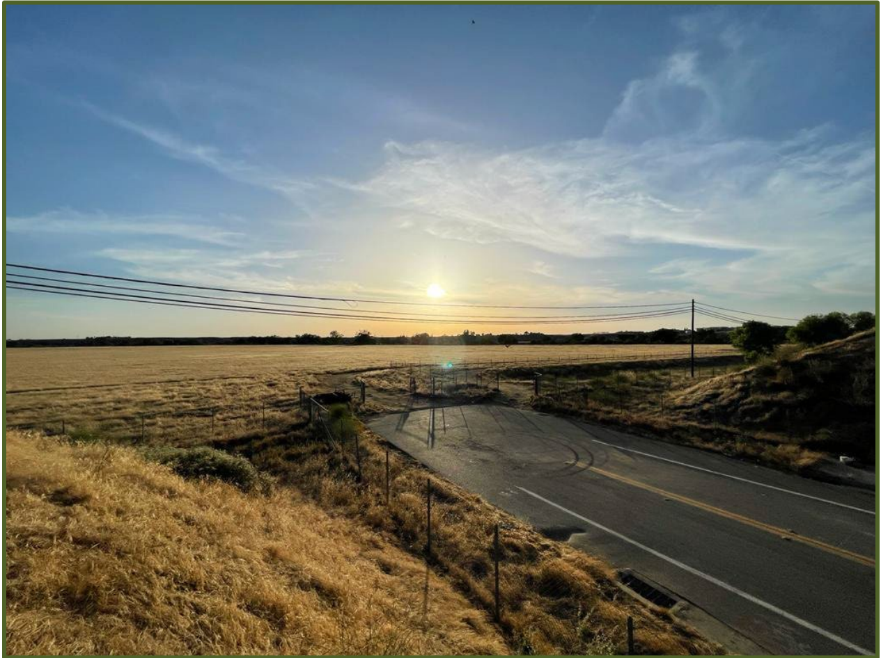
Figure 1. View facing west from existing SR 41 Undercrossing; Location of Woodward West trailhead parking
