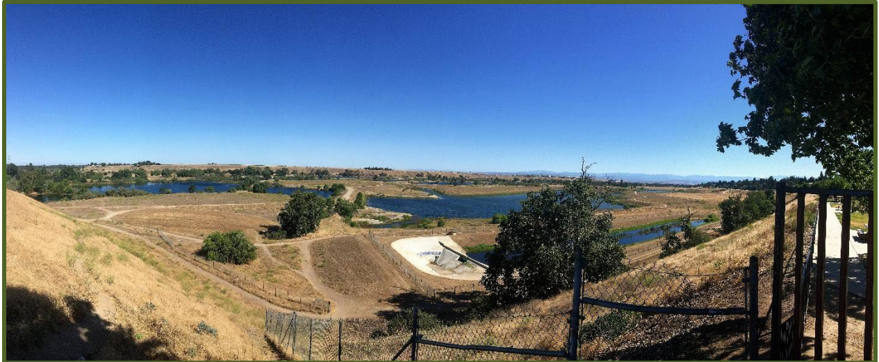
Figure 3. View facing north from corner of Spano Park where new stairway will descend bluff to Fresno River West area
